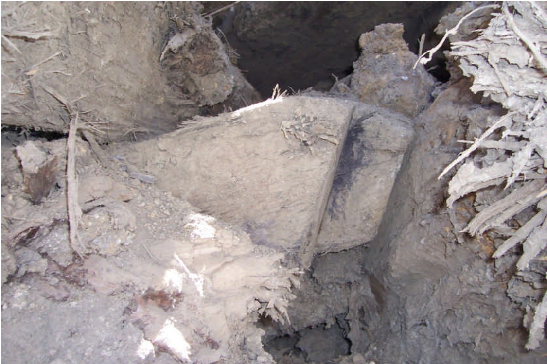
Details of several of the large timbers removed from below the stone abutment on the west end of the River Street Bridge, illustrating both a mortise and a tenon. The beam shown at bottom was set at an angle to another timber, based on the cut of its tenon, as if used as a diagonal knee brace.
