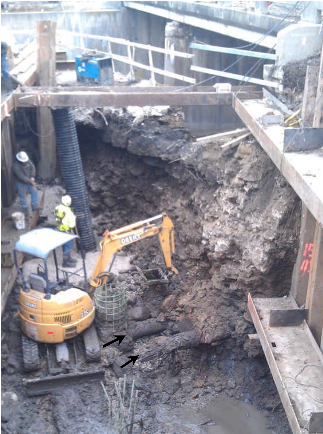
Photograph taken during the excavation of a trench along the rear side of the west end of the Blackberry Creek Dam. This excavation work exposed a line of large oak timbers extending beneath the end of the dam and the stone abutment for the River Street Bridge. Two of the timbers are marked with arrows.
