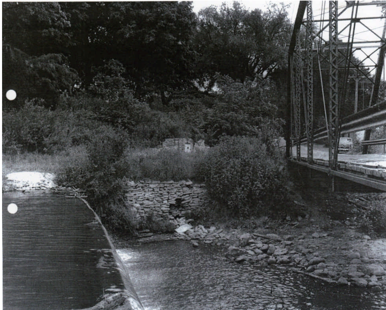
Photograph of the Blackberry Dam site, taken in 1959 prior to the replacement of the iron-truss bridge across Blackberry Creek at River Street. The fall of the dam appears at left, while the soon-to-be-replaced iron-truss bridge is shown at right. Note the dry-laid stone retaining wall between the dam and bridge. The head race for the old Blackberry Mills ran along the narrow strip of level ground between this wall the wooded bluff in background.
