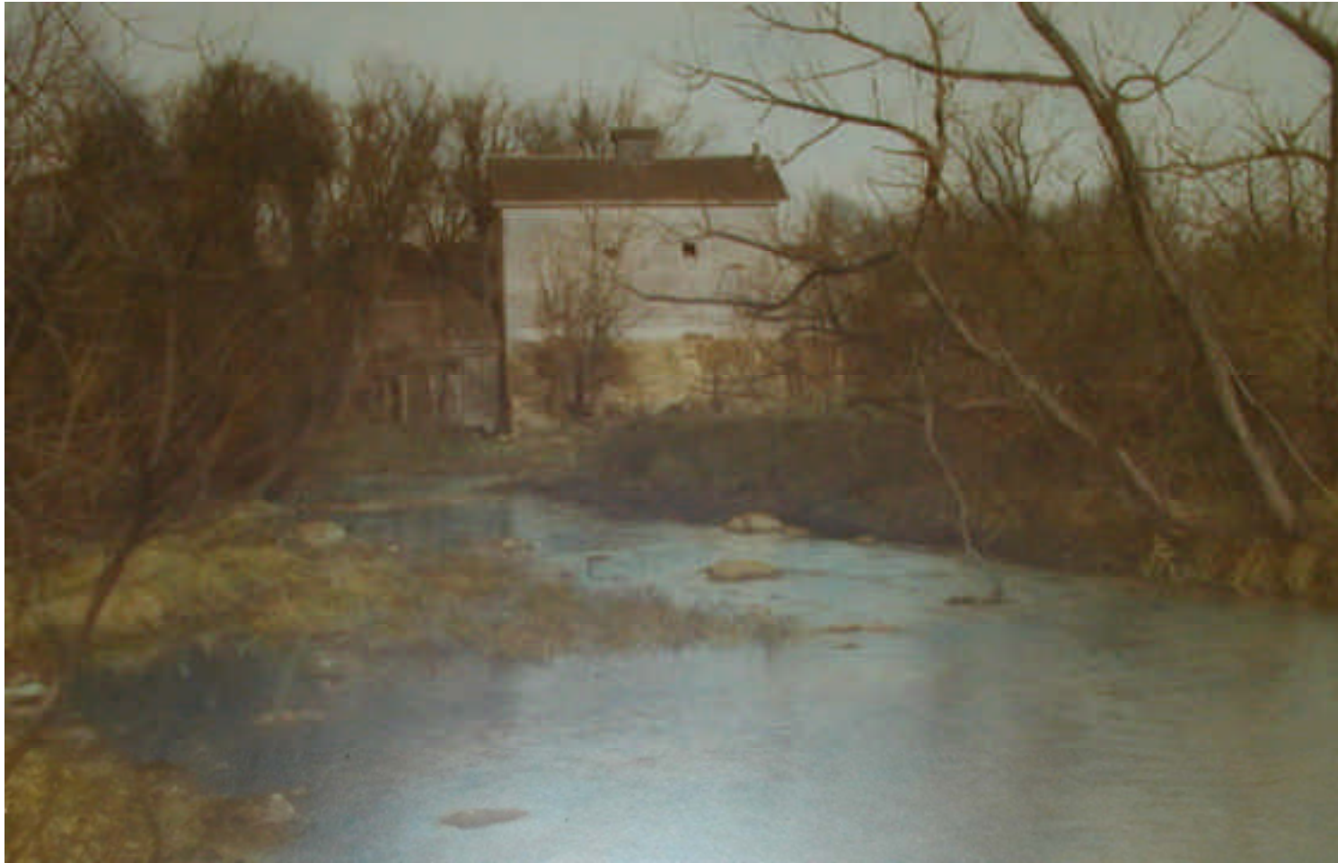
Undated painting of the Blackberry Mills, showing it as it appeared early in the twentieth century. This view looks north, up Blackberry Creek, towards the mill. The main body of the mill sits on a raised stone foundation. The lower frame section at left is the wheel house. The engine room formerly attached to the south side of the mill is not depicted and apparently had been removed some years before (based on the size of the tree shown at its former location). This painting is in the possession of the Kendall County Historical Society. This painting is in the possession of the Kendall County Historical Society. A tag attached to the painting notes that the mill had been demolished by 1936.
