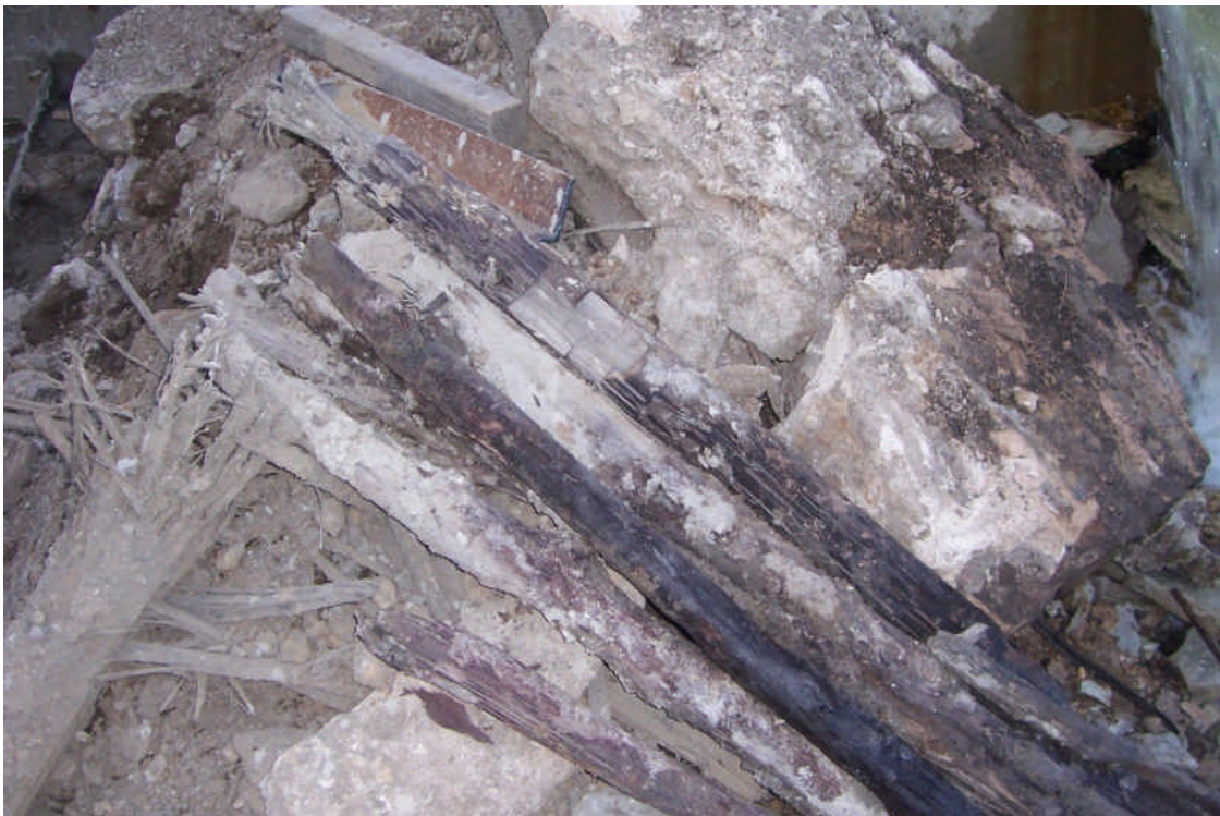
Two views of timbers found in the backfill behind the stone abutment of the River Street Bridge. These timbers left in the round and were relatively small in diameter, in contrast to those used to undershore the abutment (and illustrated in preceding figures). They were cut with an axe. They were used as fill or perhaps had been employed as a temporary work surface (for stability) during the construction of the abutment.
