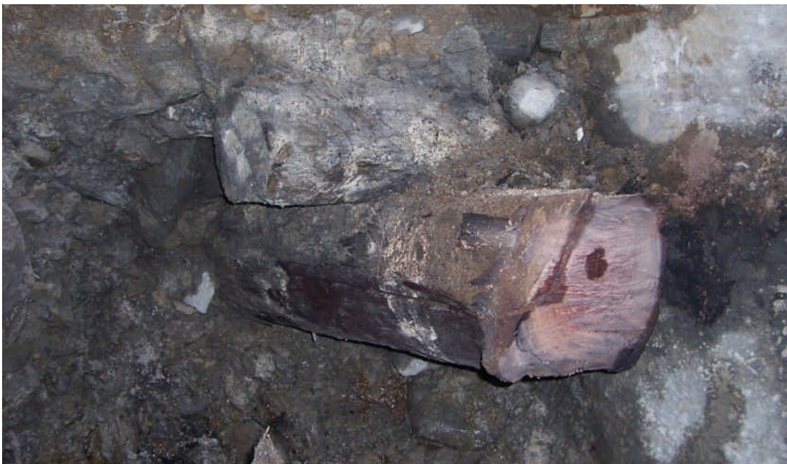
Two views of large oak timbers found in situ beneath and behind the stone abutment on the west end of the River Street Bridge. (TOP) Row of timbers set parallel to the stone abutment, with arrows indicating individual members. The dashed line indicates the juncture between the dam and abutment. Note that a number of the timbers are located beneath the west end of the dam as well. (BOTTOM) Timber projecting out from the excavation trench behind the stone bridge abutment. This was located behind and perpendicular to the abutment.
