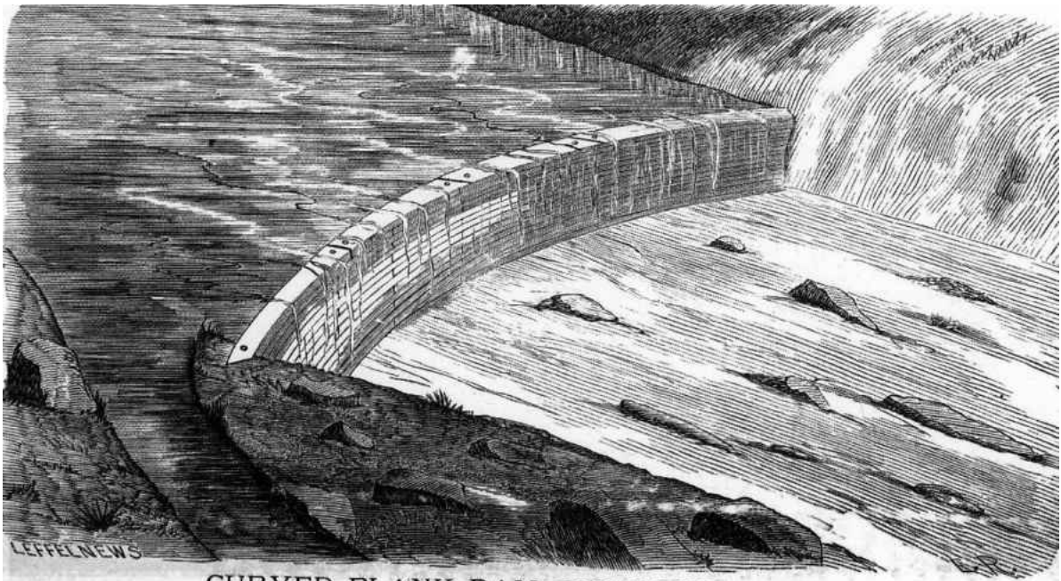
CURVED PLANK DAM FOR ROCK BOTTOM.
