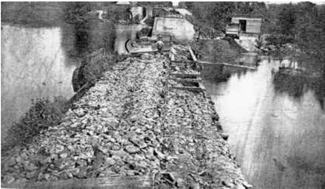
Two 1930s-era photographs of the low-water feeder across the Du page River at Channahon, Grundy County, Illinois. This was a cribbed dam built to raise the river level so that water would be directed into the section of the Illinois and Michigan Canal extending west of Chamahon. (TOP) View of the dam prior to its rebuilding by the Civilian Conservation Corps. Note the planking covering the top of the dam. (BOTTOM) View of the dam after the removal of its top planking, showing its underlying timber cribbing and stone ballast. The cribbing for the dam appears to have been three sections wide.
